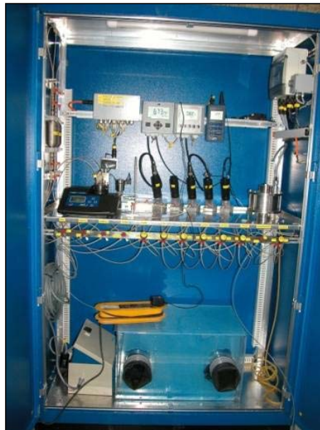
Extraction flow control and analysis
