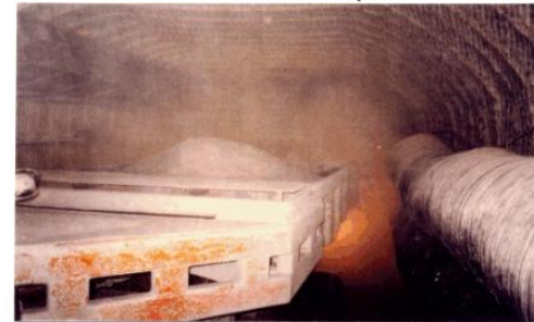
Backfilling Slinger Truck in a Disposal Drift
